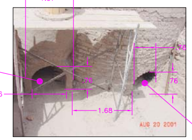
UNDER GROUND TUNNEL DETAIL ELEVATION VIEW 10K SCALE 1"= 40'
